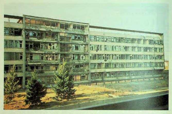
Figure 1. Eastern view of the northern part of the main building of the Vinkovci Medical Center. Beside broken windows, a more careful inspection reveals numerous large-caliber hits.
