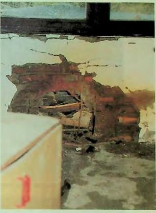
Figure 4. Damaged outer wall of the Pediatric Ward room on the first floor.
