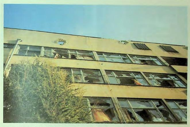
Figure 2. Western view of the southern part of the main building of the Vinkovci Medical Center. Beside broken windows, holes made by direct shell-hits are visible.
