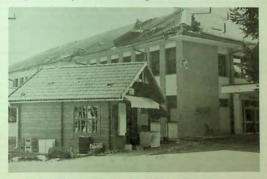
Figure 5. Damaged facade and the roof of the new Outpatient Building.
