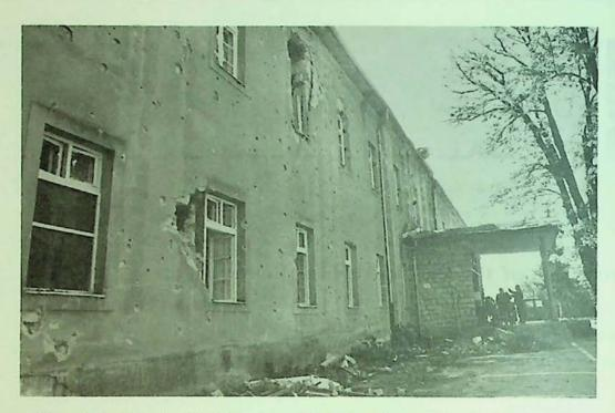
Figure 1. Facade of the old building, damaged by bullets and pierced by artillery shells.
