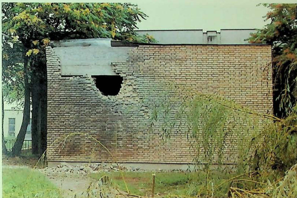
Figure 10. Canteen damaged by a rocket from a multiple rocket launcher.
